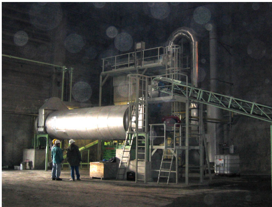
Picture 6: view of the SEROX drying facility of ALSA Hannover
