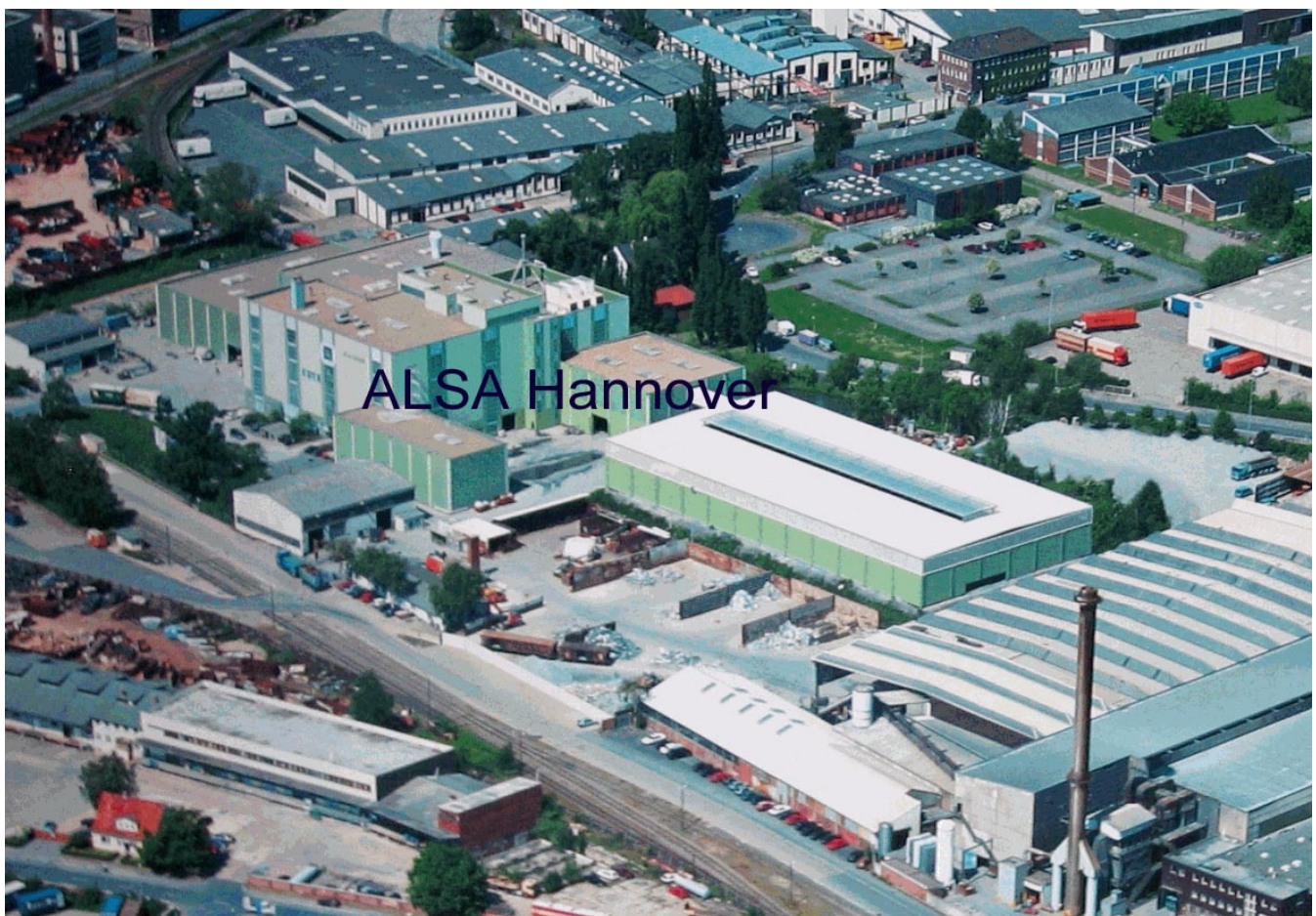
Picture 3: ALSA's treatment facility at Hannover/ Germany
